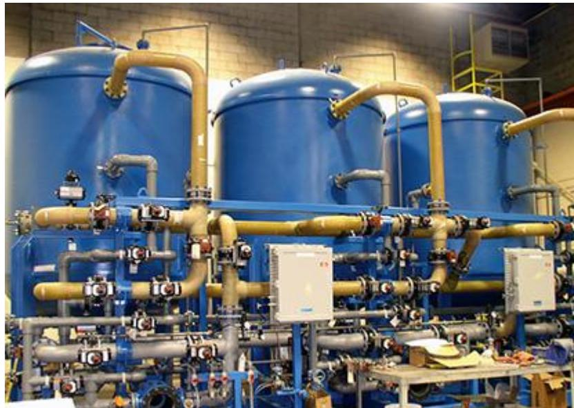
Ion exchange reactions are stoichiometric, (i.e., predictable based on chemical relationships) and reversible. The strategy employed in using this technology is to exchange somewhat harmless ions (e.g., hydrogen and hydroxyl ions), located on the resin, for ions of interest in the solution (e.g., regulated metals). In the most basic sense, ion exchange materials are classified as either cationic or anionic and in that way they are similar to other solution phase reactions. For example:
